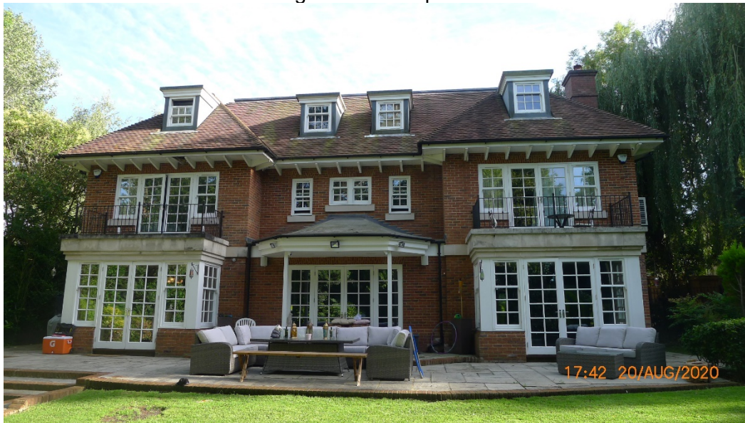
Figure 2: Rear elevation of the existing house
